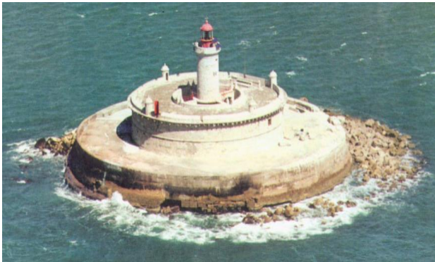
Figure 5: Bugio Lighthouse in 1993, before the reconstruction work. Photo courtesy, Eng.º Lopes de Castro.
