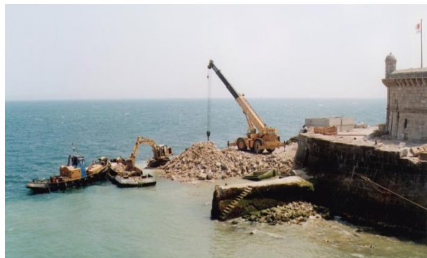
Figure 8: Bugio Lighthouse in 1998. Placement of Antifer cubes. Photo courtesy, Eng.º Lopes de Castro.
